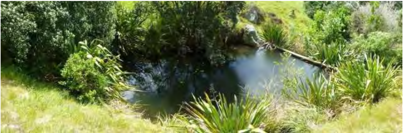
Figure 14: Panoramic view of Lower Emergency Landing Dam
