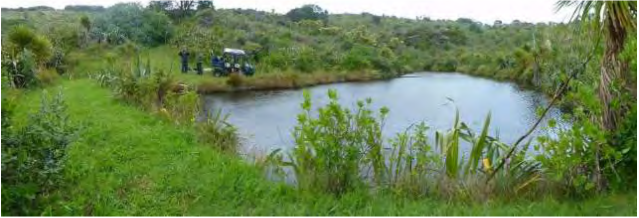
Figure 28: Panoramic view of Lower Silvester Dam
