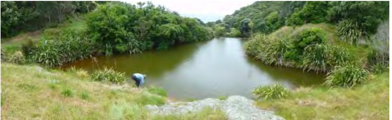
Figure 8: Panoramic view of Upper Emergency Landing Dam
