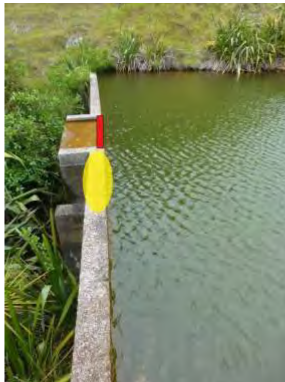
Figure 61: Area of spillway to be blocked off (red bar) and section of dam wall to be lowered (yellow highlight)
