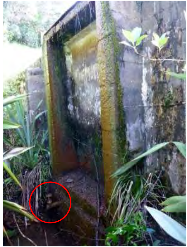
Figure 10: Base of spillway structure, showing drainage valve (circled)
