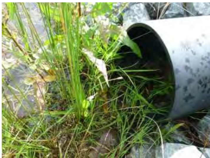
Figure 25: Outflow pipe for Upper Silvester Dam
