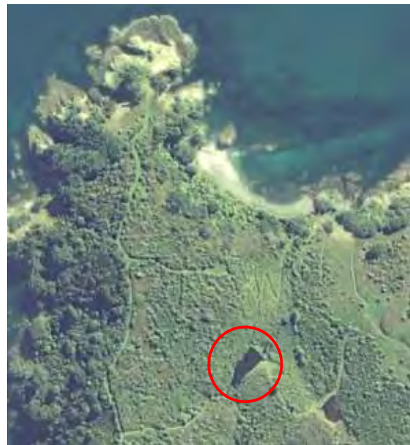
Figure 27: Aerial view of Lower Silvester Dam
